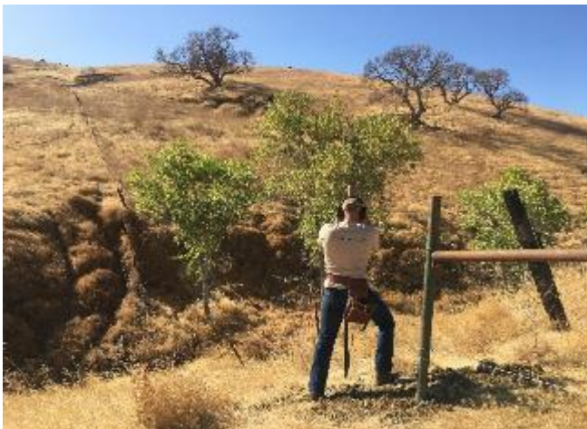
Installation of H-brace for fencing (Dash)
