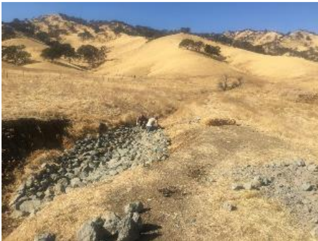
Riprap placement in main drainage ditch (Dash and Olivia) Removal and maintenance of pump (Dash and Olivia)
