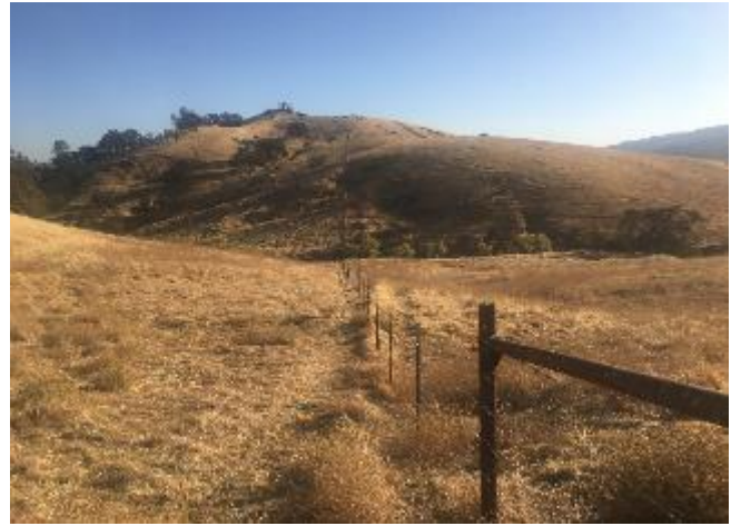
Completed fencing on East side of field
